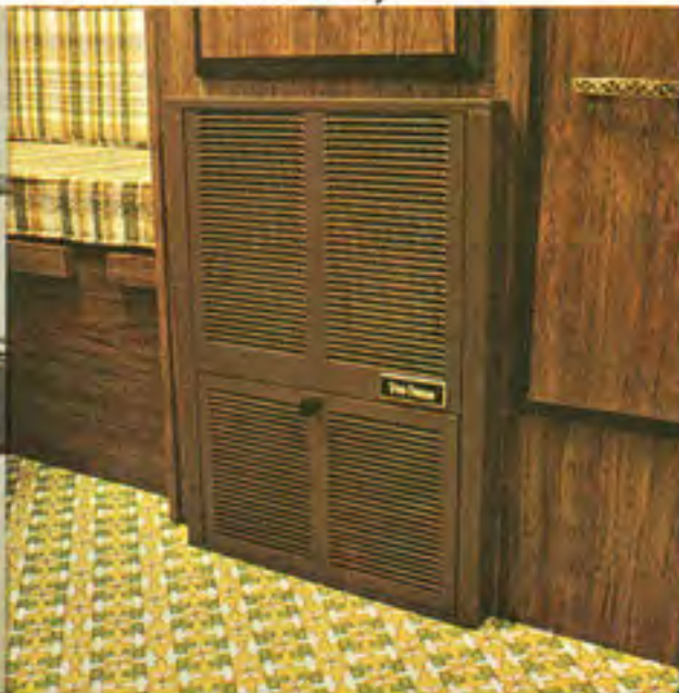
Fresh air vented heater. (9,000 BTU on Starlite, Starmasters & Stardusts—11,000 BTU on all Galaxies.)
